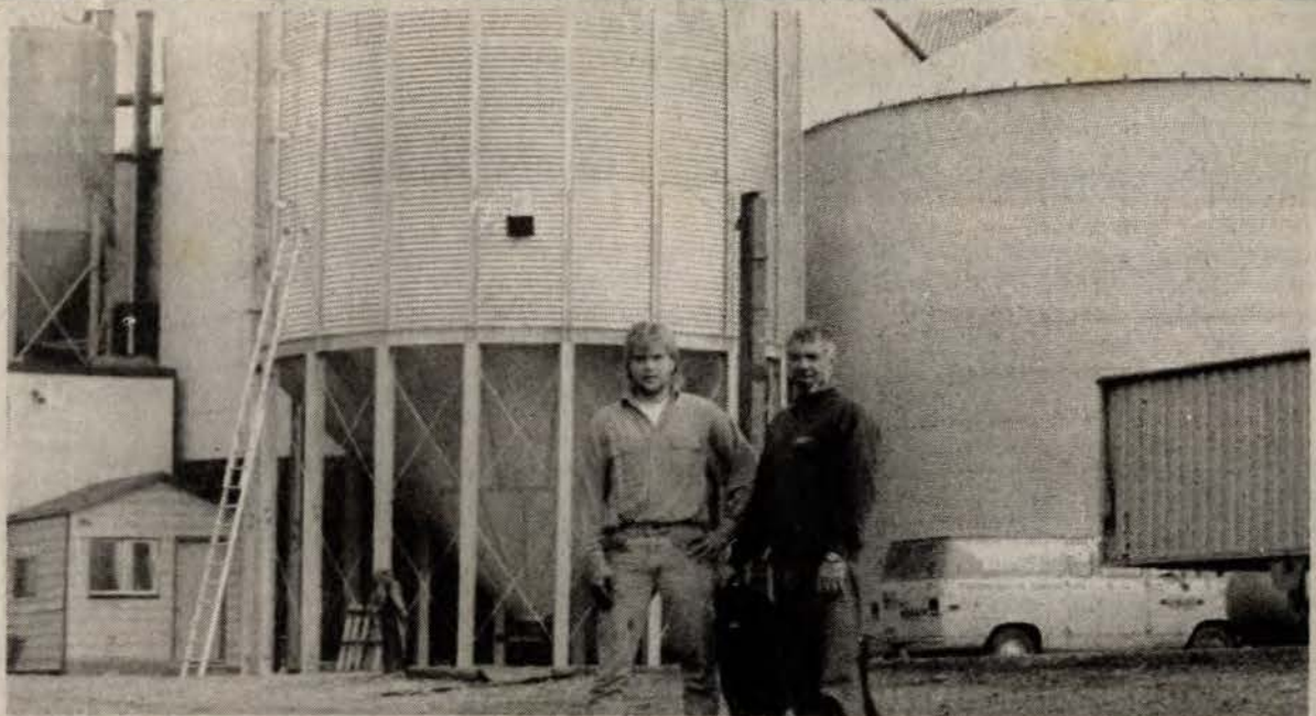
BUSY PLACE — Gerry Vanderwyst, son of Paul and labrador Caesar are framed by the newly-constructed grain elevators at Vanderwyst Brothers, RR 7 Aylmer. —(Staff)
